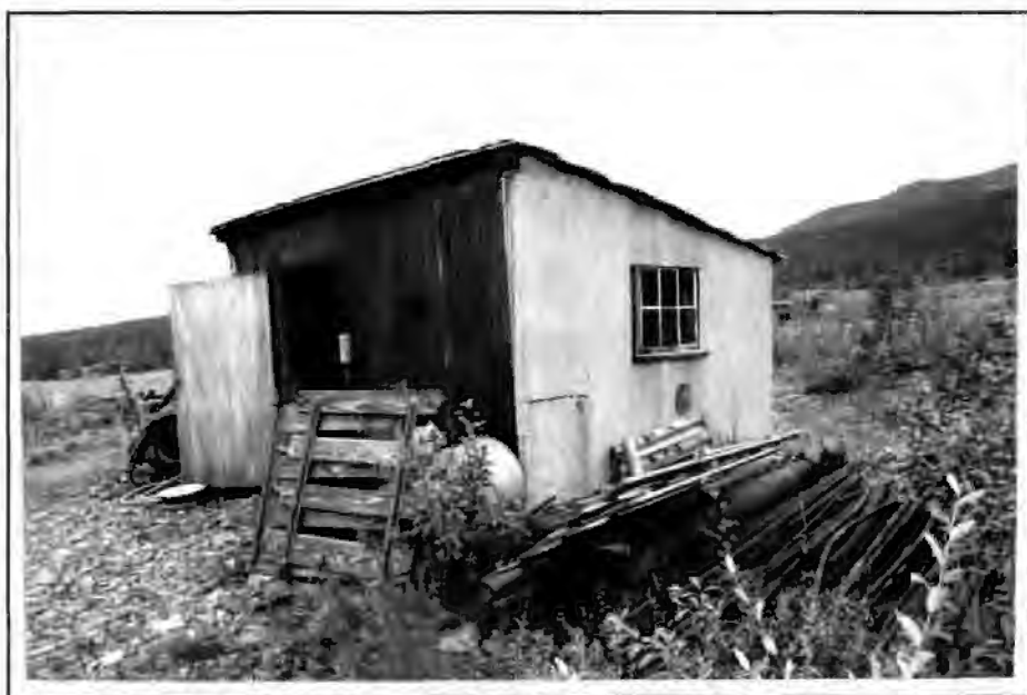
Figure 145. The Fuel Storage Shed, 1993. The view is looking southeast.
